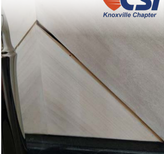
Tongue and groove wood paneling gap showing unfinished surfaces
