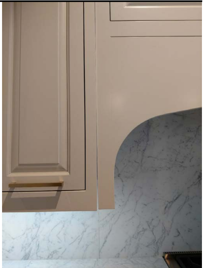
Cabinet work separated due to shrinkage
